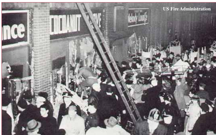
The Cocoanut Grove nightclub fire in Boston in 1942, which killed 492 people, led to strict standards on emergency egress and fire protection centered on the use of hinged swinging doors.
