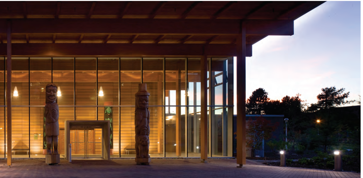
A view of the First People's House at the University of Victoria in British Columbia, Canada, designed by Alfred Waugh Architect.
